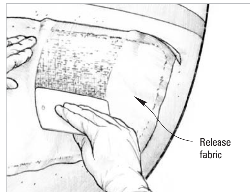
Figure 4-6 Squeegee over the release fabric with firm pressure to remove excess epoxy and smooth the patch.
